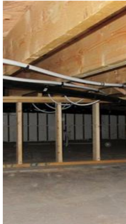
Renovating Old Homes
