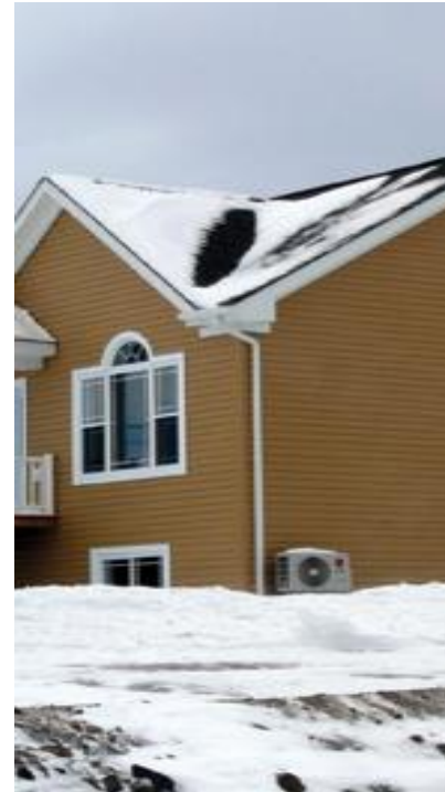
Building New Homes
