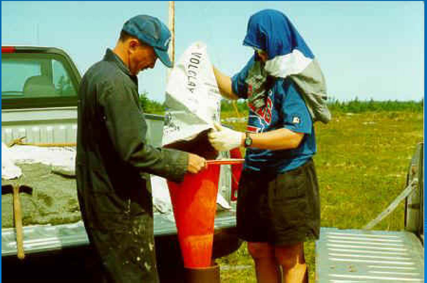
Sealing / Decommissioning a well
