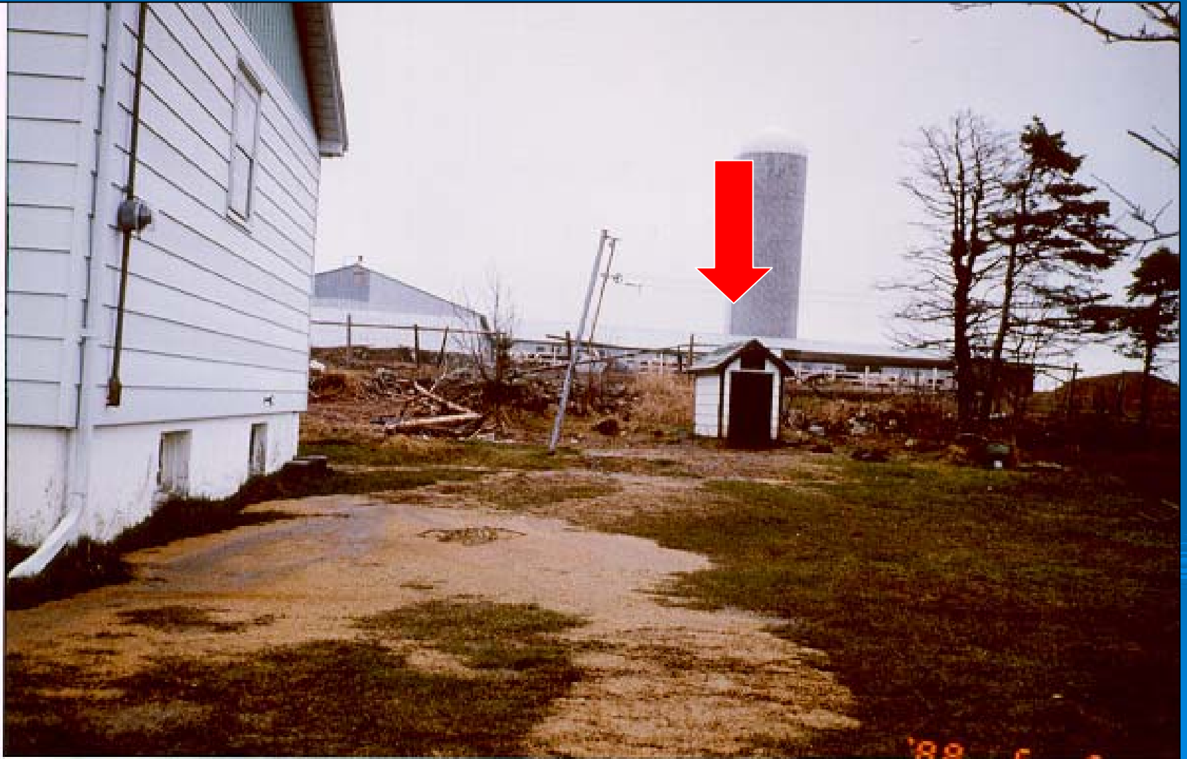
Improper Location of Farm and Private Well Showing Farm Runoff
